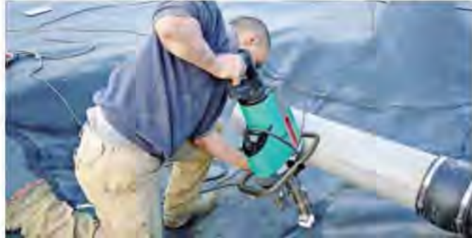
WELDPLAST S6 undertaking assembly applications on a landfills site.
