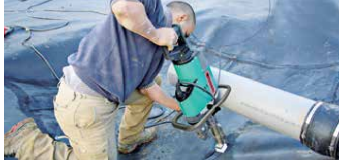
WELDPLAST S6 undertaking assembly applications on a landfills site.
