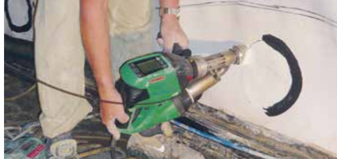
The robust WELDPLAST S2 welding a patch in a tunneling application.
